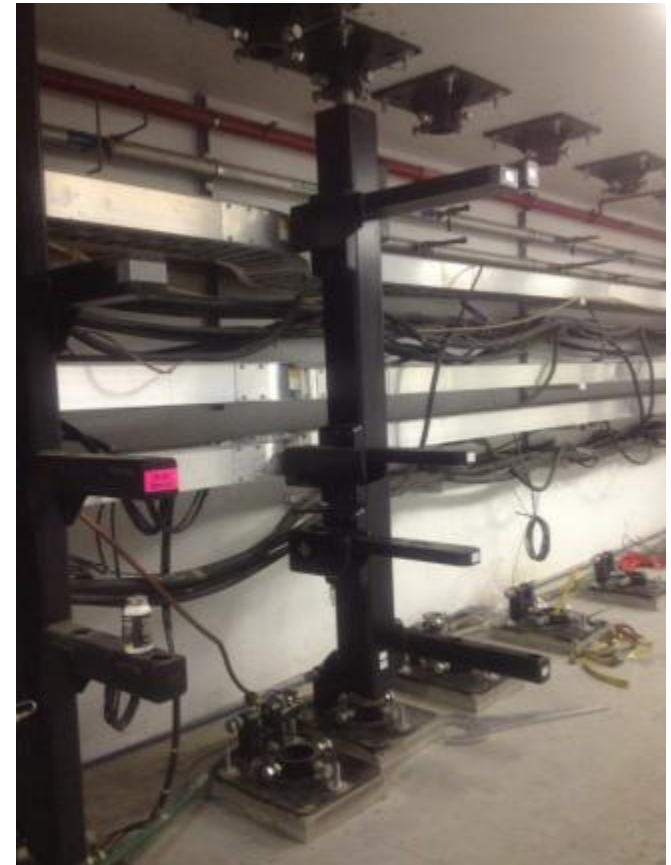
Stand installation: 1R+
