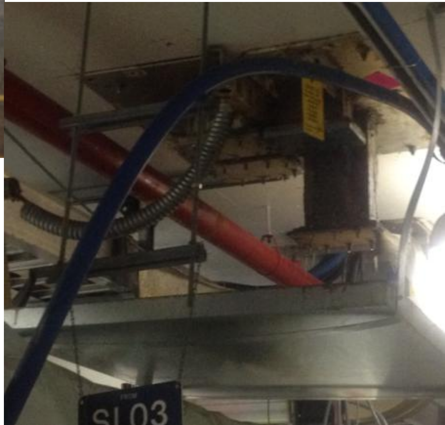
2L03 WG penetration repair
